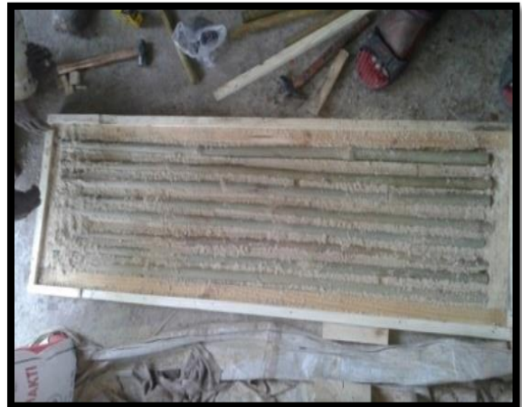
Fig 8(e): Preparation of Bamboo Panel
