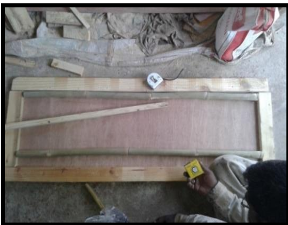
Fig 8(b): Preparation of Bamboo Panel
